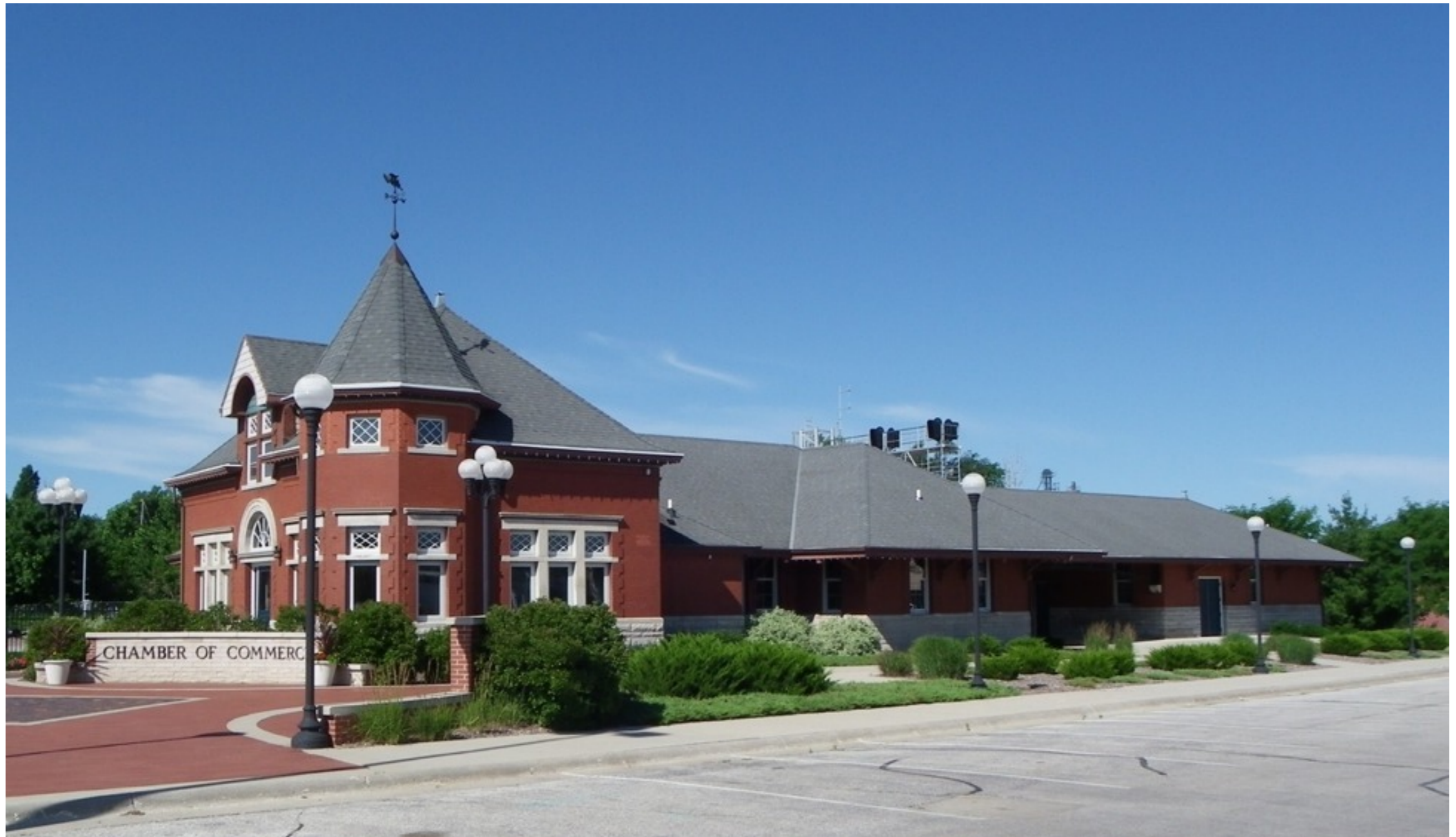
Full length view of the main depot structure.
