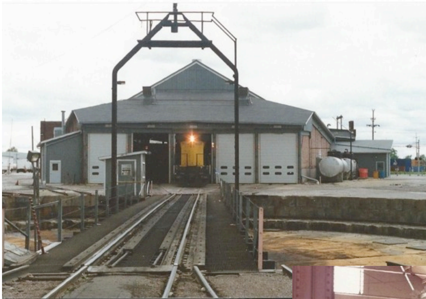
North side of roundhouse with turntable bridge and pit area. (05-30-93).
