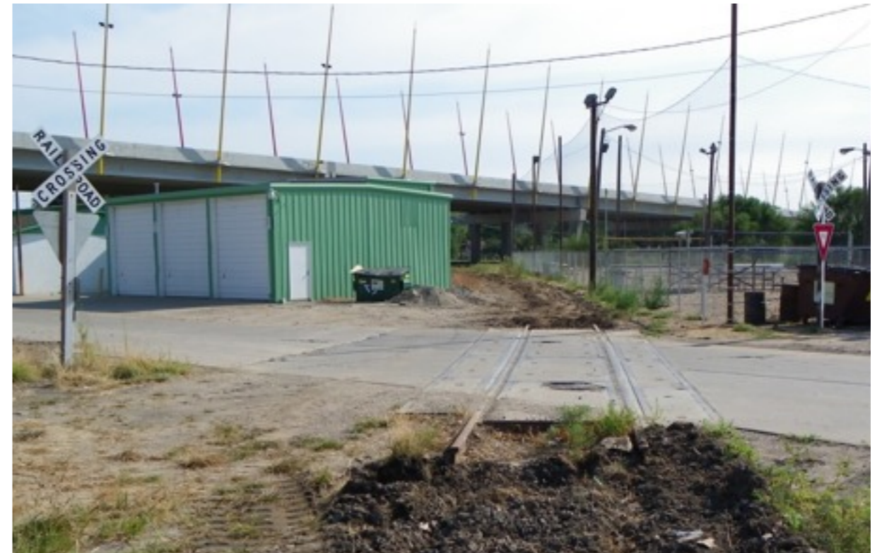
12 th Street crossing looking east.
