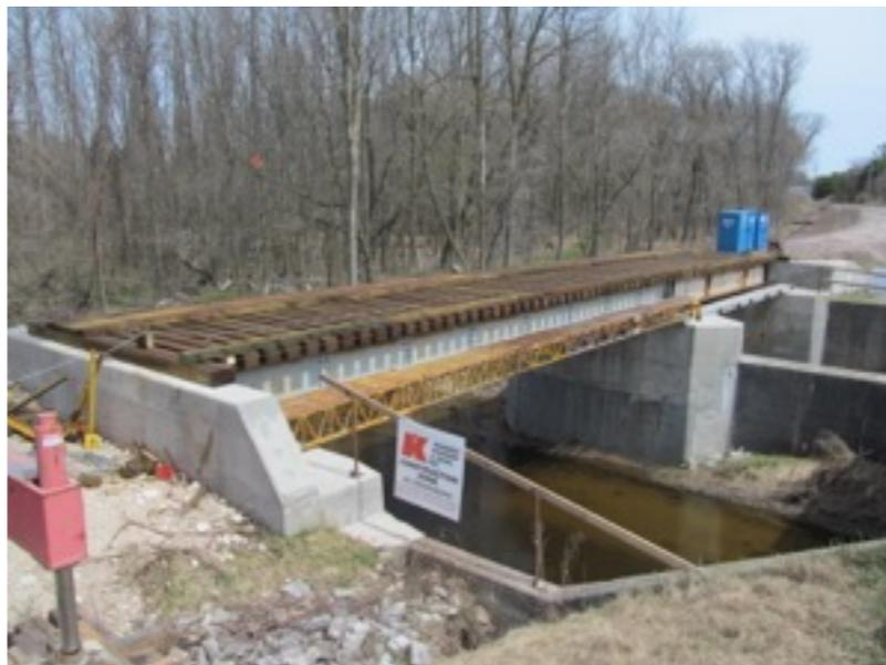
**Bridge over the Mullet River along Co. Hwy. PP:** They installed the brand new deck timber on top of the support beams. It looks like the deck is nearly complete ready for rails to be attached some day. Photos #3 & #4.
