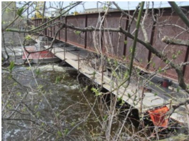
**Bridge over the Sheboygan River - Downtown Sheboygan Falls:** Seems most of the work is being done to the support beams and the center pier of the bridge. The photo looking through some branches at the underside of the bridge, gives an overview of the temporary work platform under the bridge. (Someone should trim those branches before the leaves pop out!!)
