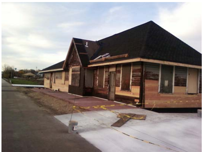
Replacement of rotted siding is under way
