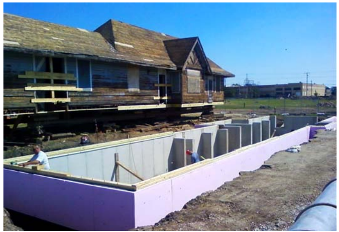
Workmen put on the finishing touches
