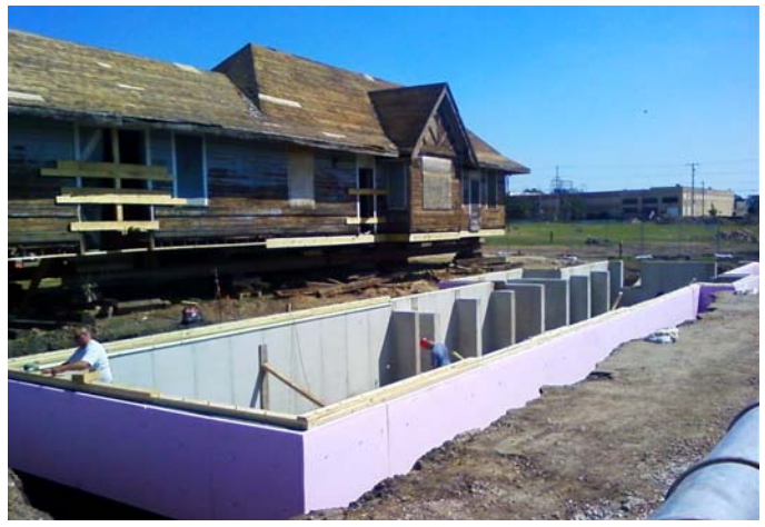
Workmen put on the finishing touches
