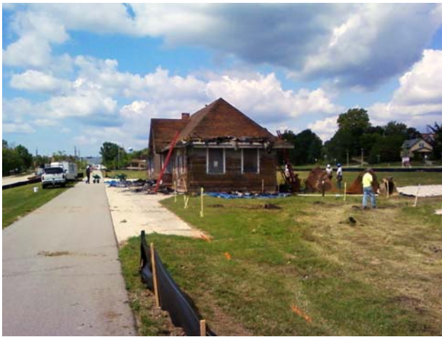
Old shingles and asbestos are removed from the depot
