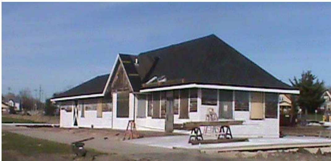
Old shingles and asbestos are removed from the depot
