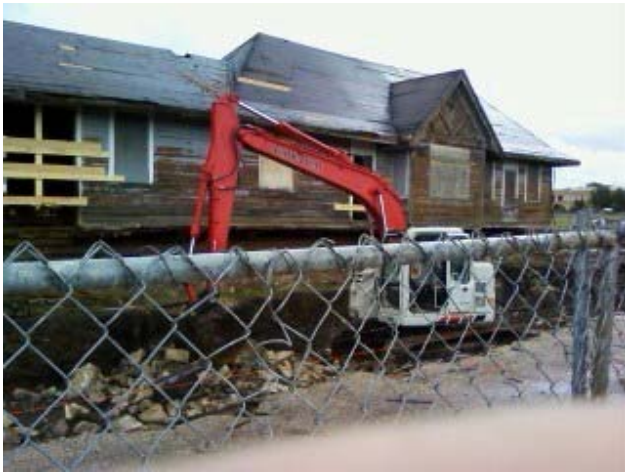
Digging the new basement
